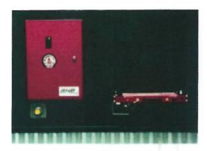
Our storage vault is equipped with automatic 24-hour fire detection with an Ecaro25 fire suppression system (pictured below). No water based fire suppression is utilized in the vault. Our Ecaro25 based clean agent fire suppression system meets all ANSI, ISO & NFPA requirements.
