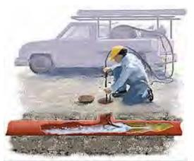
Municipalities can hire professional plumbing services to remove trapped sediment and debris from storm drains with periodical flushing (Source: Drain Patrol, no date)
